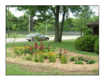
recharging groundwater and removing stormwater pollutants. The garden's flat bottom helps distribute rain water evenly across the planted area. Topsoil amended with compost and sand allows the water to slowly soak into the ground within a few days so there is no standing water to breed mosquitoes.
