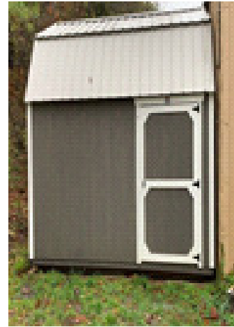
Addition on back for storage
